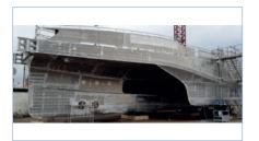
A hull during construction, showing the opening in the centre hull that allows for greatly reduced waterplane area in SWATH mode
